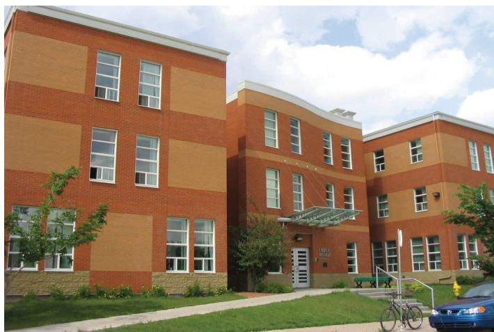
This project typifies homeless funding excesses. Moving from a 62 bed rental bldg with a $600K/year budget into a brand new architecturally designed $4 million 75 bed shelter industry owned bldg with a $900K/year budget and adding only 13 very expensive beds.
